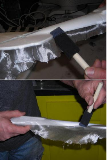
Work slowly around tight curves, the cloth will conform to surprisingly complex surfaces. Cut cloth if/when necessary to fit into corners.
