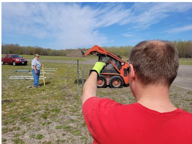
Brian Johnson makes sure the posts are in line.
