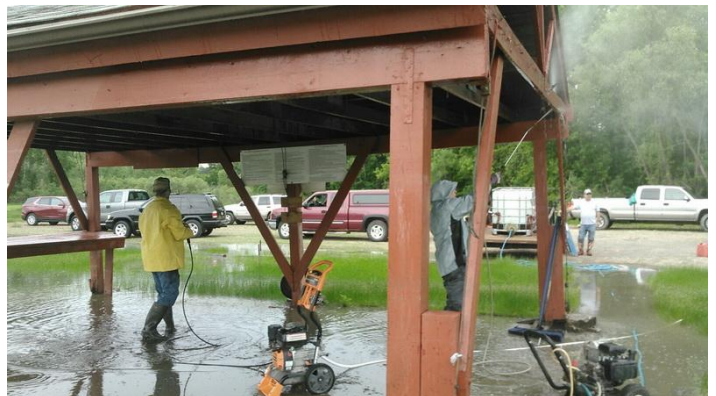
The shelter starts to look pretty good.
