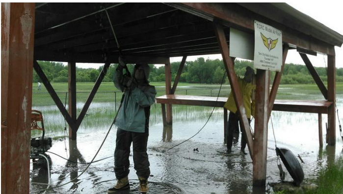
High pressure action in the rafters of the shelter.
