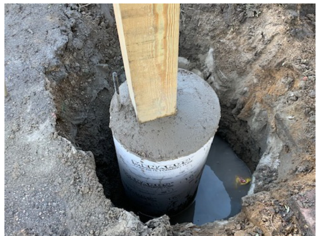
The new footing is poured around the post.
