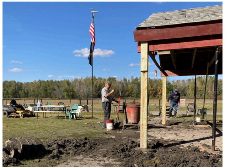
Two posts replaced! (Photo by Tom Hall)
