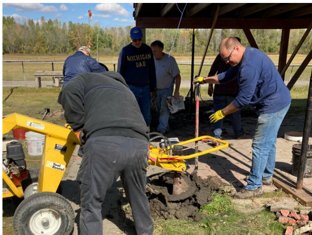
Using the power auger to deepen the hole.
