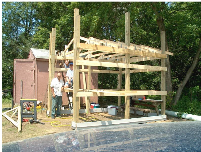
Jim R, John D and Rick Smith framing the shed. Photos by Jim Ronhovde
