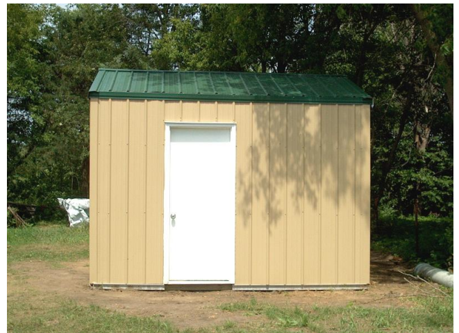
The new TCRC tractor shed almost done.
