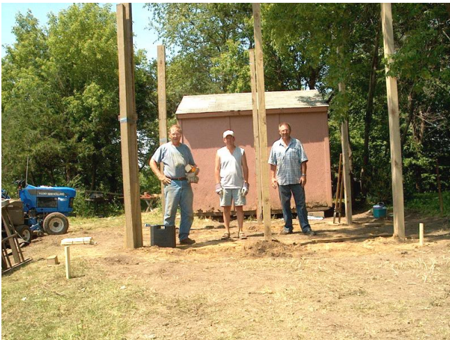
John Dietz, Dave Erickson & Jim Ronhovde set the corner posts for the new shed.
