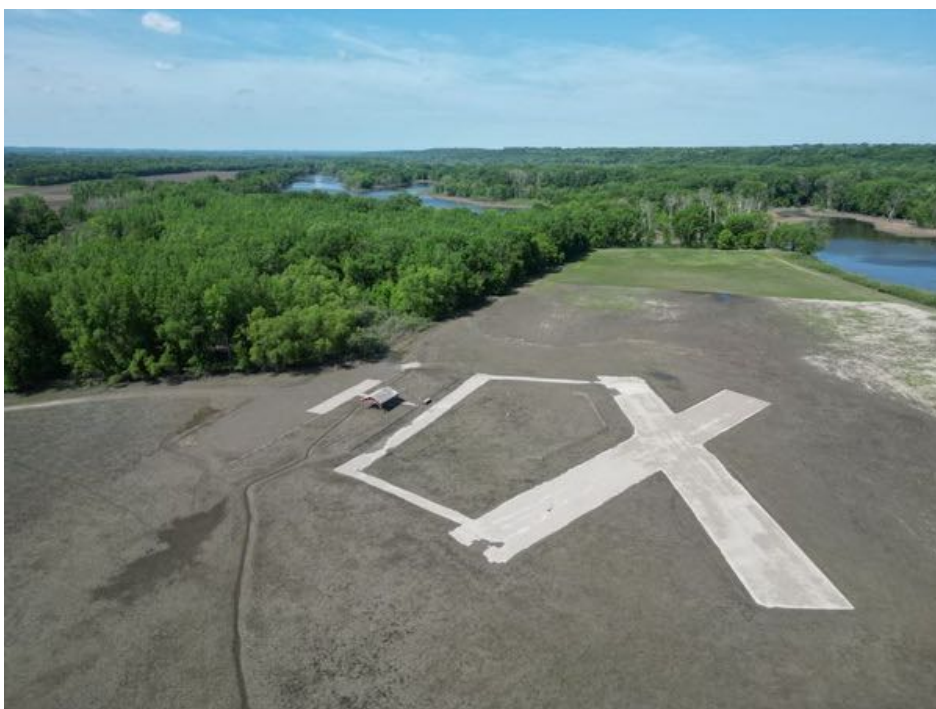
The runways, taxiways, pits, shelter, parking lot and road are free of the Minnesota River. (Drone photo by Dick Voeltz)
