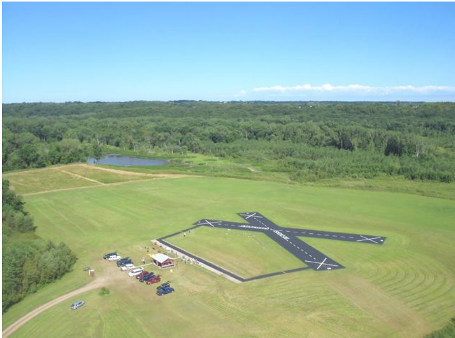
The TCRC runways look great from the air after being seal coated and striped. (Photo by Jay Bickford)
