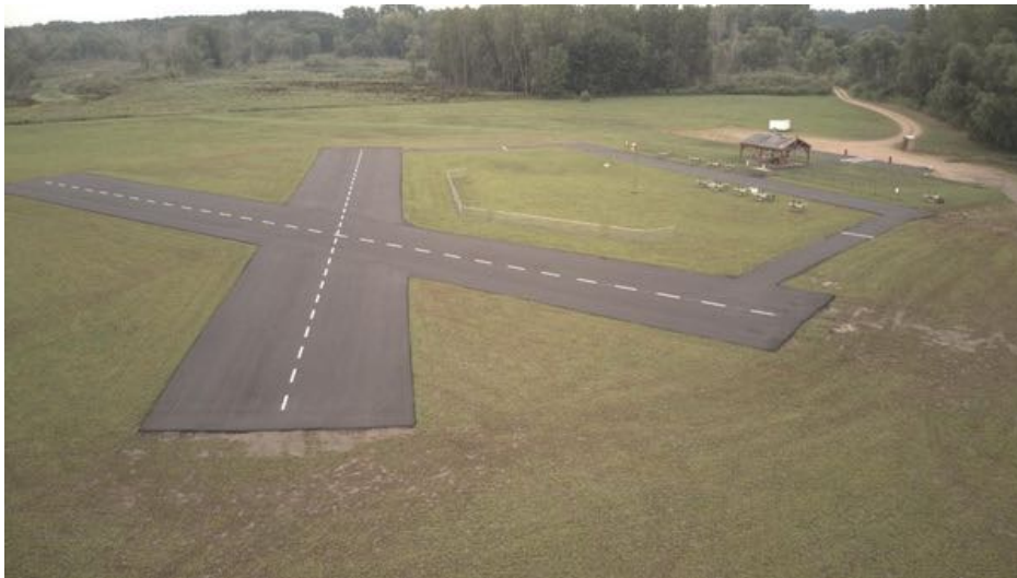
An aerial view of the total project completed, including the addition of the centerlines on the runways. What a great looking field! (Aerial Photo by Richard Voeltz)
