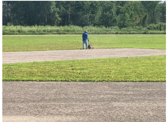
It was a lot of surface area on the runways that had to be swept and readied for the new surface.
