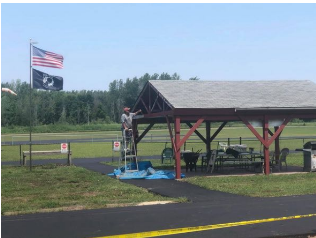
Mark Wolf finishing up the shelter painting.
