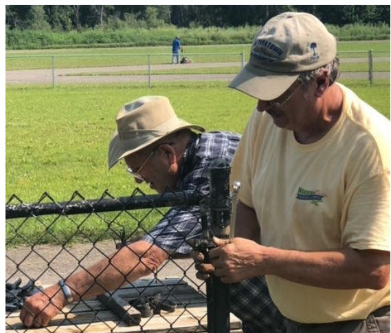
The chainlink fence got some work also.
