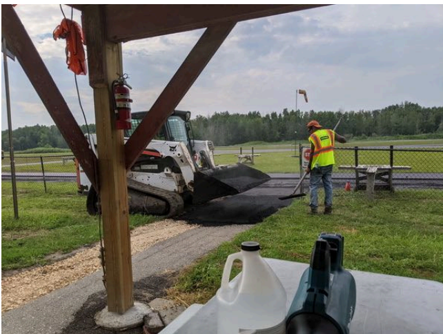
Paving the sidewalk by the shelter.
